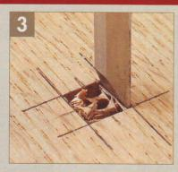
Now, cut with the grain to square off the remaining edges of the mortise. The intersecting edges of the mortise have already been established, so this part of the cut will go smoothly.
